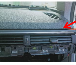
19. Pry out the central air conditioning panel
